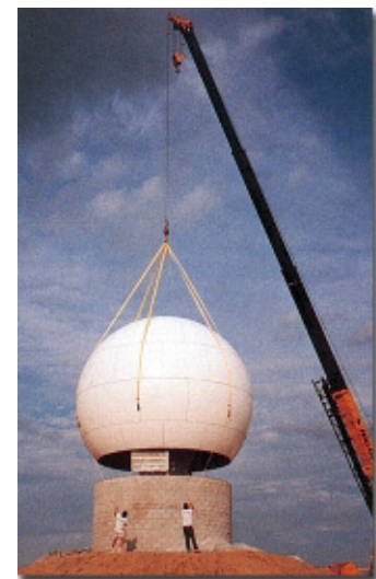
Strong, lightweight FRP/Composite domes use self-supporting sandwich construction to protect sensitive electronic equipment from the Sabara to Antarctica while remaining transparent to the electromagnetic signals.
