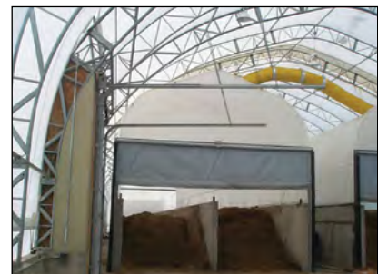
Photo 5-25: Channel composting system © Scott Gamble
