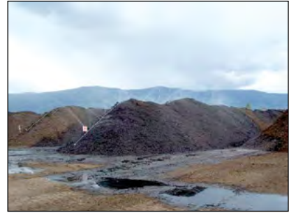
Photo 5-4: Water can be added to windrows and stockpiles using sprinklers © CH2M HILL
