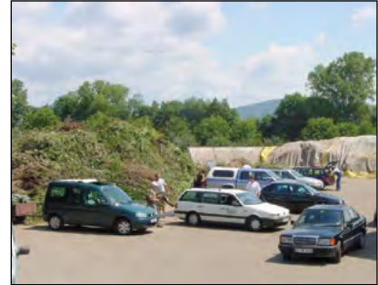
Photo 10-1: Multiple, clearly defined unloading positions should be provided, especially at facilities that cater to residential customers © Scott Gamble
