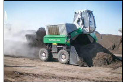
Photo 3-6: Turning windrows with a front-end loader or windrow turner reintroduces oxygen and re-establishes porosity © CH2M HILL
