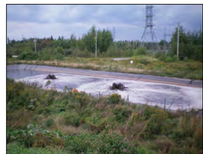
Photo 10-9: Contaminated stormwater is commonly collected in retention ponds and is reused in the treatment process © CH2M HILL
