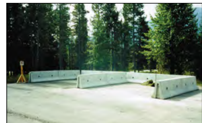
Photo 5-6: Small bunker composting system © Scott Gamble
