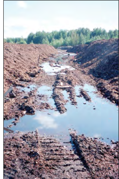
Photo 15-8: Rutted surfaces limit access, attract insects, and are a source of odour © CH2M HILL
