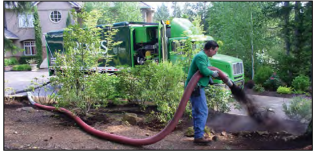
Photo 17-1: Blower trucks are commonly used to place or spread compost for erosion control applications © Rexius Forest By-Products Inc.
