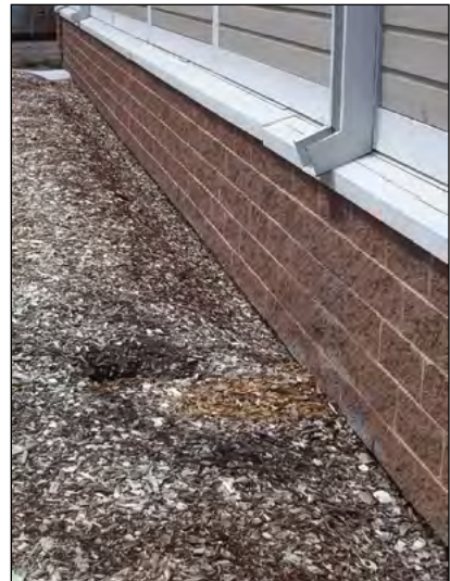
Photo 10-11: Water from roof drains should be directed around operating areas to minimize the quantity of contaminated surface water that has to be collected and treated © Scott Gamble
