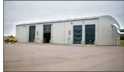
Photo 10-3: Engineered steel frame receiving building © CH2M HILL
