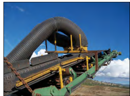
Photo 15-5: Vacuum systems can be used to remove litter from material on conveyor belts © CH2M HILL
