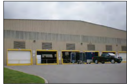
Photo 9-11: Waste management facility with receiving doors for self-haul traffic that are completely separated from the doors used by larger waste collection vehicles © CH2M HILL
