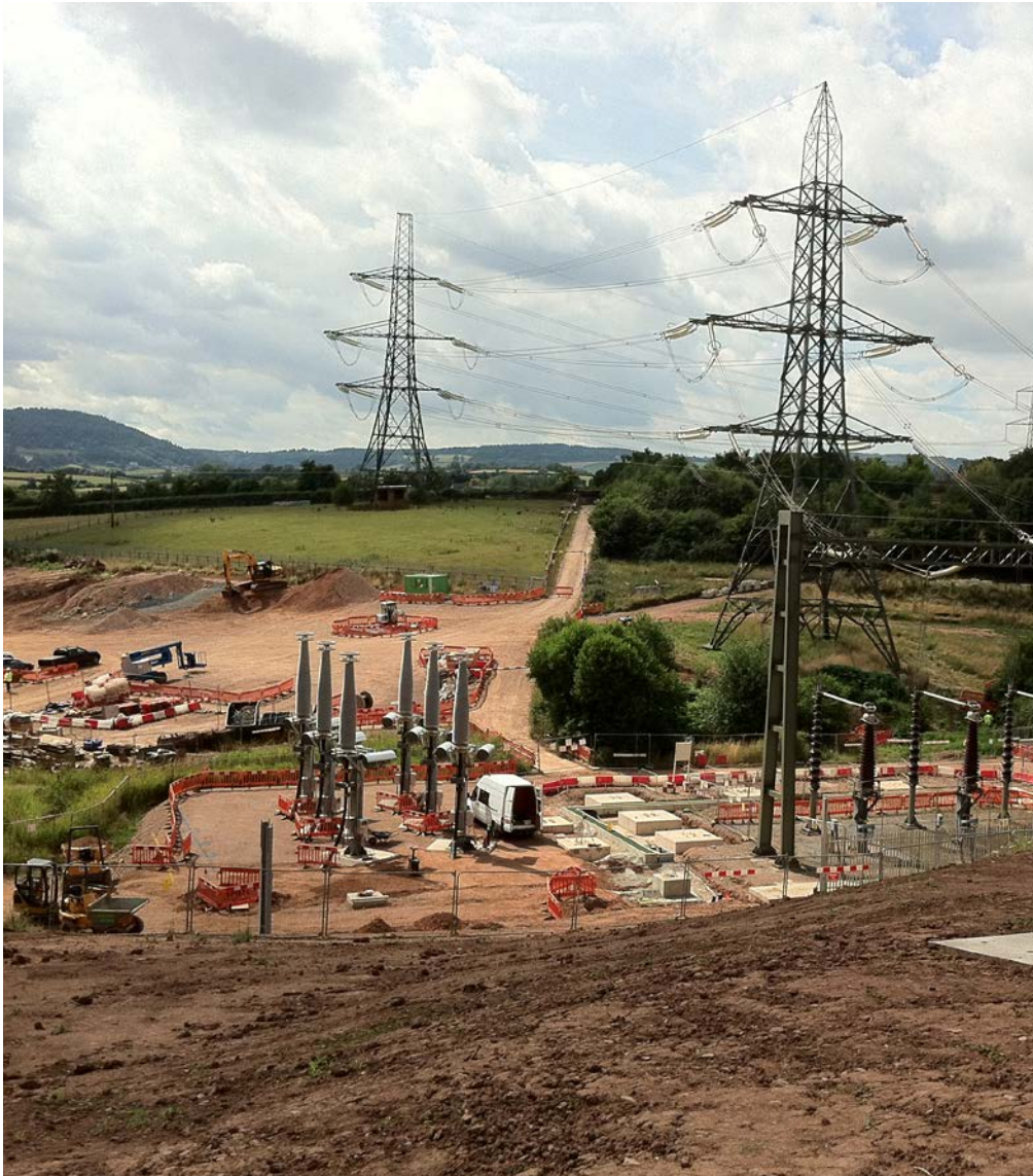
The undergrounding of electricity cables at Ross-on-Wye
