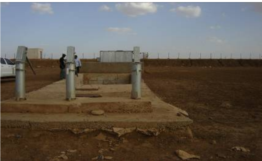
Figure 2. Slow sand filtration system under construction for the hafir at Dar Hashay, Kassala State
