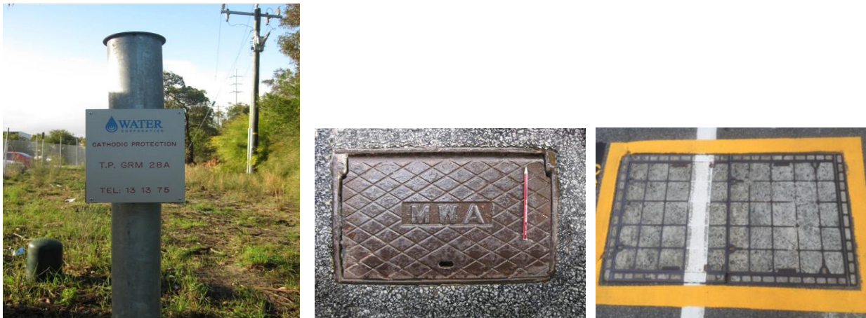
Figure 1 Cathodic protection test point (left); valve cover; trafficable sewer maintenance cover
