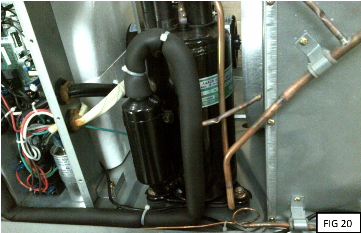
View of Compressor inside Rooftop Unit
