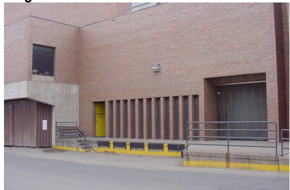
Rear Facade (Stage Door/Loading Dock)
