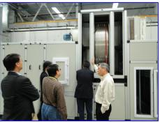
Installation of Desiccant Wheel inside the Air Handling Unit
