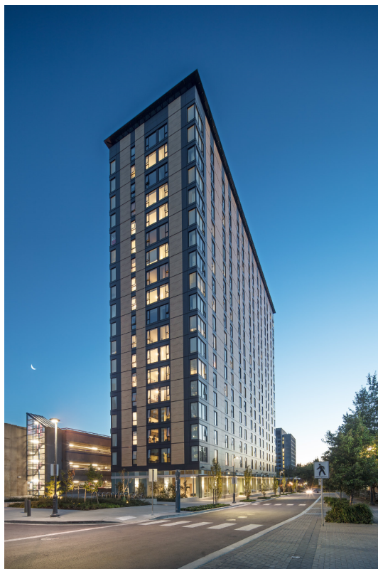
Fig. 14. Brock Commons, an 18-story student residence building at the University of British Columbia, was the world's tallest wooden skyscraper when completed in May 2017. Image CC BY-NC 2.0 University of British Columbia.
