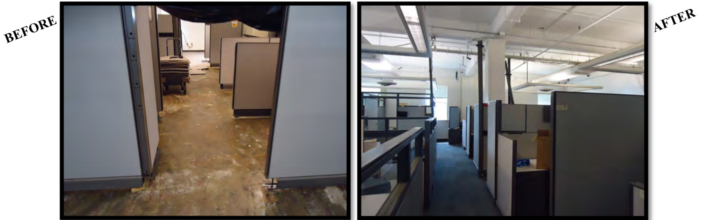
Daly Hall Renovation
