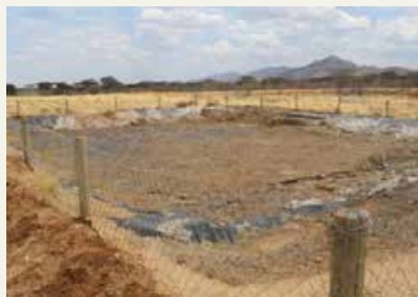
Figure 10: An exposed waste disposal area
