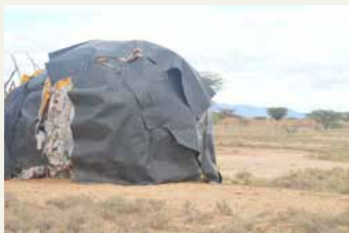
Figure 9: Showing some waste PVC used as roof cover for manyatta
