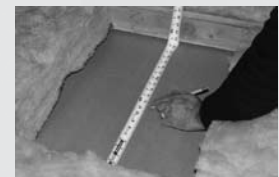
Inside attic fig. 2
