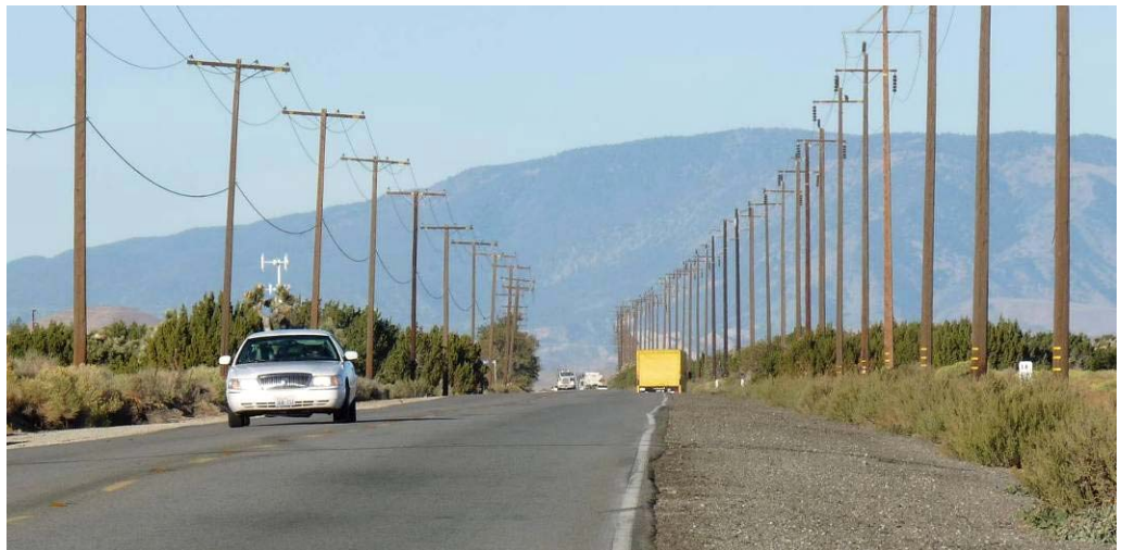
Figure 2.1. The LA138 test road on Highway 138 in the Mojave Desert.
