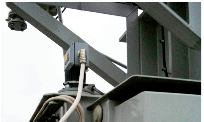
Temperature switch monitoring internal oil temperatures
