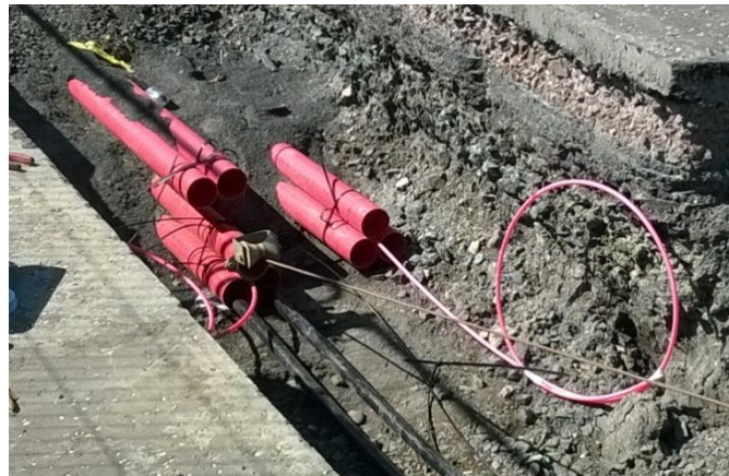
Figure 9: Shared trench with three circuits
