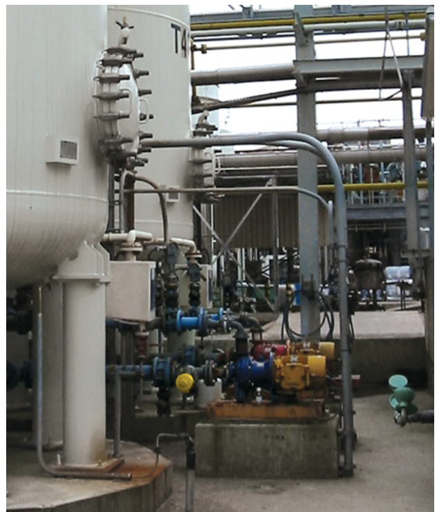
Figure 1: FCI Model FLT93S flow/level switch protects pumps from dry-run and other operational downtime conditions
