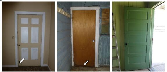
Various conditions of exterior doors- crack at north door, rot at south door, east door in good condition (NPS Photos 2013)
