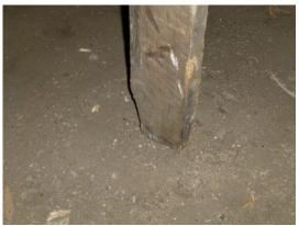
Eccentrically loaded pier footing at centerline of building and column in connection with dirt. (NPS Photos 2013)
