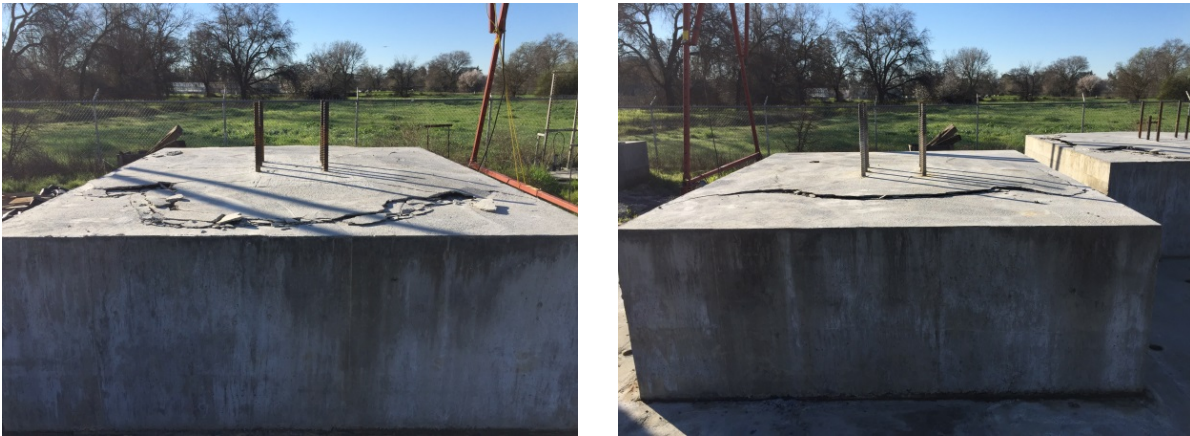
Figure 6 – Profile view of breakout surface for (a) 12-inch embedment and (b) 18-inch embedment
