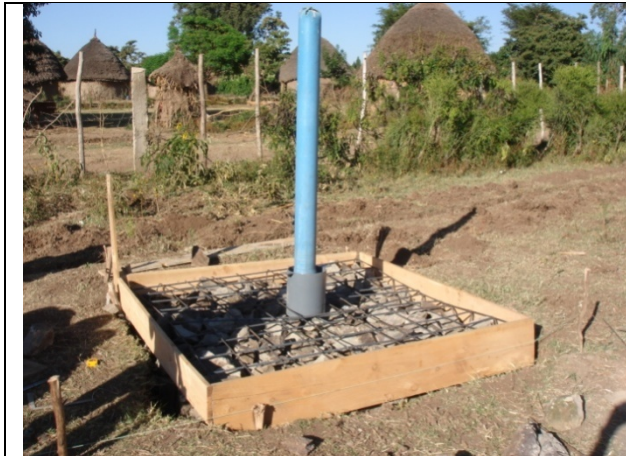
Construction concrete base for well head
