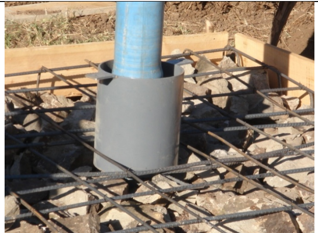
Incorporating well head into concrete base
