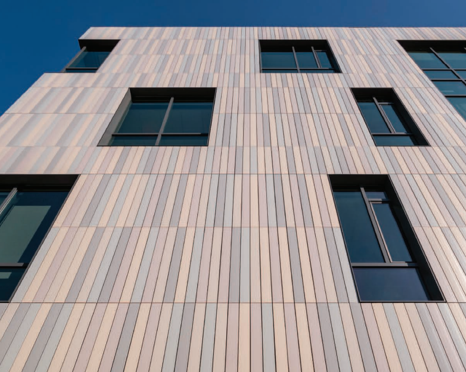
Tykeson Hall (top) employs terra cotta with open-joints (bottom right) and five color glazes on a neutral clay body. We looked at similar glazing methods like Mayan tetrapod jar production, 200 B.C.–A.D. 1, Izalco Usulután ceramic innovation with orange on a cream-colored clay for a two-color technique with a burnished surface.
