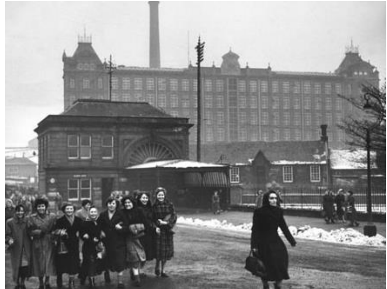
Coats Ferguslie Mill no.1 est. 1826 - demolished 1992)
