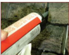
10. For a final finish, use Texture Plus® color-matched caulk to fill all screw holes and any gaps.
