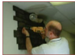
7. Screw into wall using drywall screws or finishing nails. For best look, place them in grout lines or crevices.
