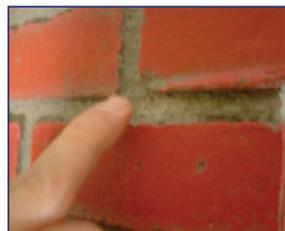
For a final finish, use Texture Plus® color-matched caulk to fill all screw holes and any gaps.
