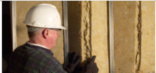
After conventional installation of steel studs and one layer of dry-wall, installer inserts 25 in. wide Creased 3-in. THERMAFIBER SAFB into 24-in. wide stud cavity, then slits blankets to a depth of about 1 in. Sound performance is completed through application of gypsum panels.
