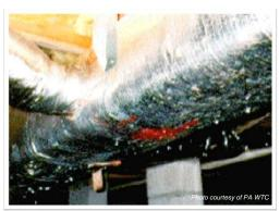
Water droplets of condensation on AC ducts.
