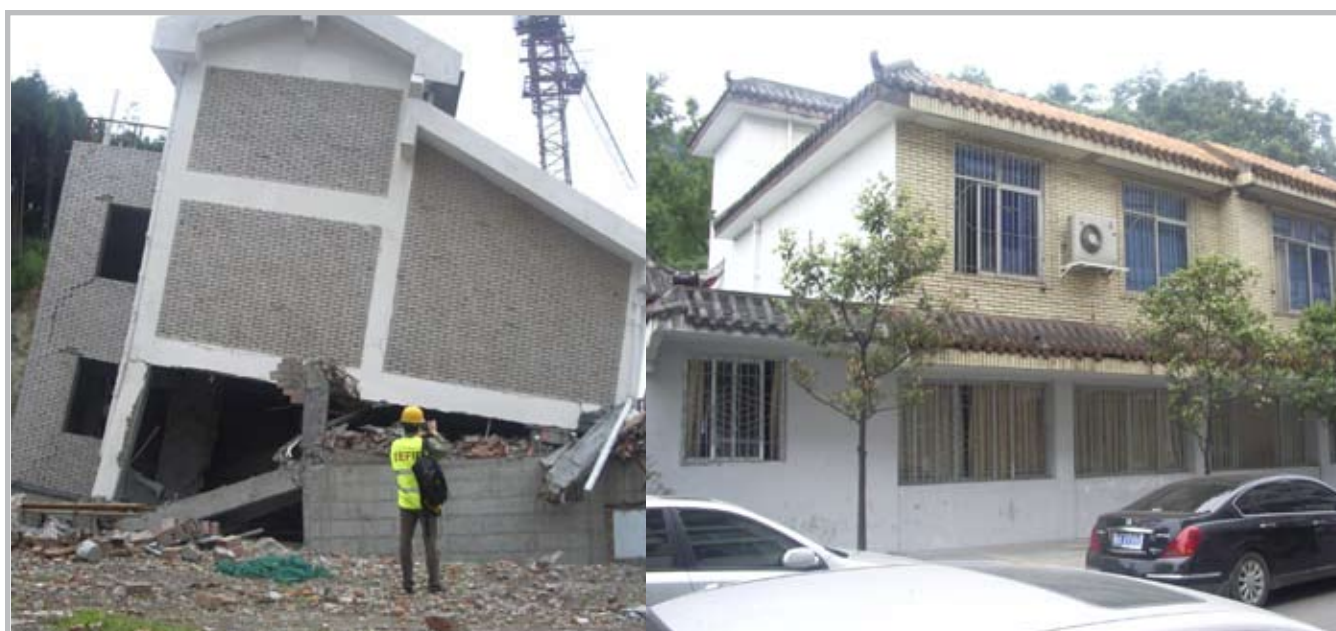
Similar buildings performed differently during the earthquake due to the type of soil on which they were constructed: the building built on rock (left) collapsed, while the building built on softer soil (right) was virtually undamaged. (Source: EEFIT)
