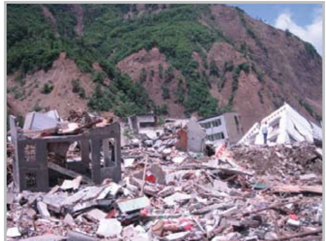
Damage to buildings in Wenchuan (Source: IEM)
