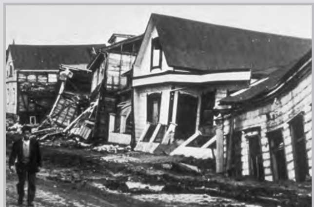
Damage to wood frame dwellings in Valdivia, Chile, following the May 22, 1960 Chile Earthquake (Source: National Aeronautics and Space Administration)
