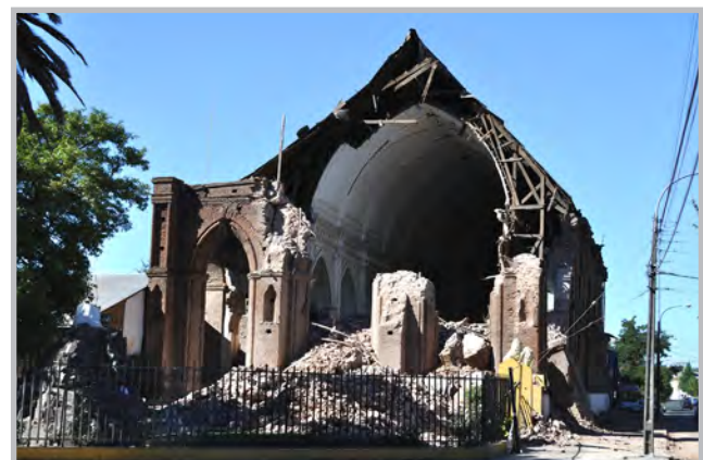
Damage to a historic church in Curicó, Chile: collapse of the Iglesia San Francisco's front tower and entrance (Source: RMS)
