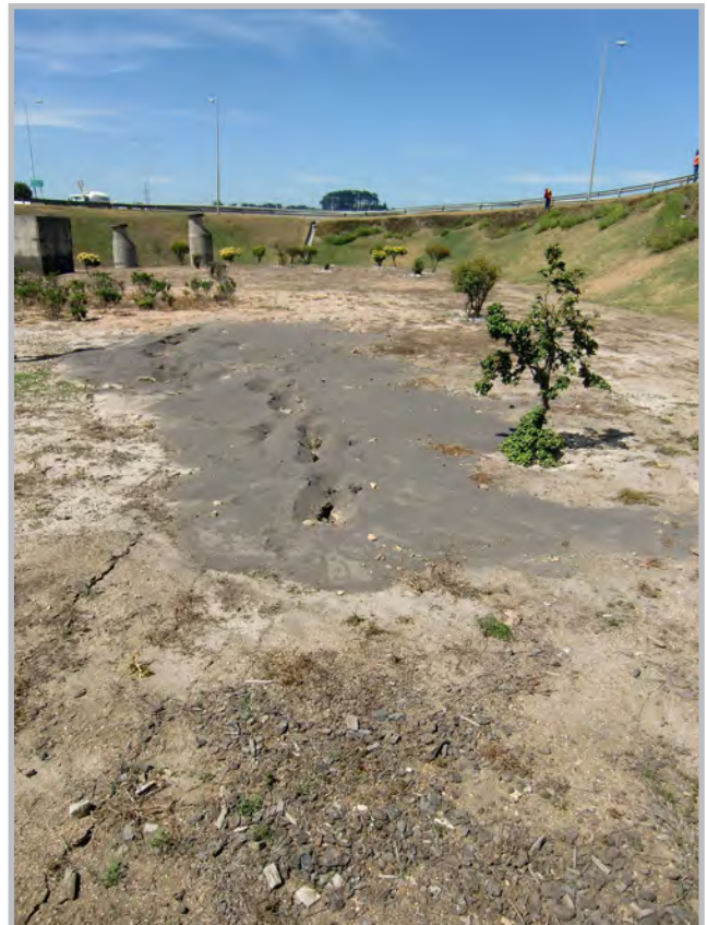
Evidence of liquefaction (sand boils) near the Juan Pablo II Bridge, which spans the Biobío River and connects Concepción to San Pedro de la Paz (Source: RMS)
