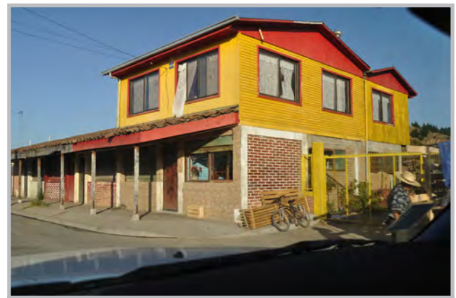
Confined masonry building in Coelemu, Chile (Source: RMS)
