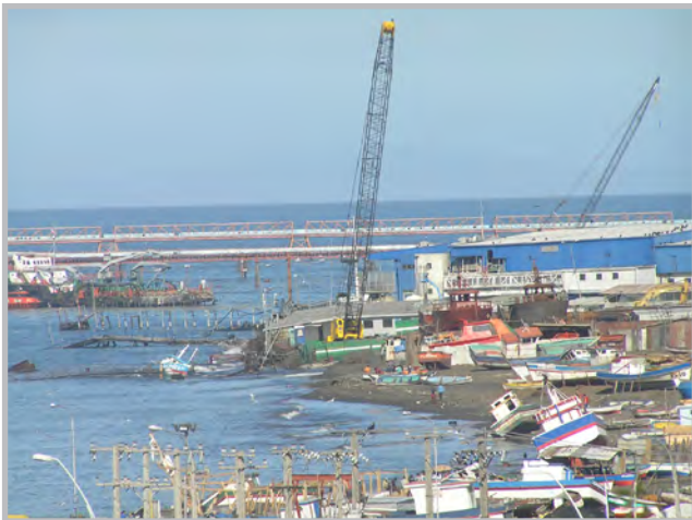
Damage to the port in Coronel, Chile (Source: RMS)
