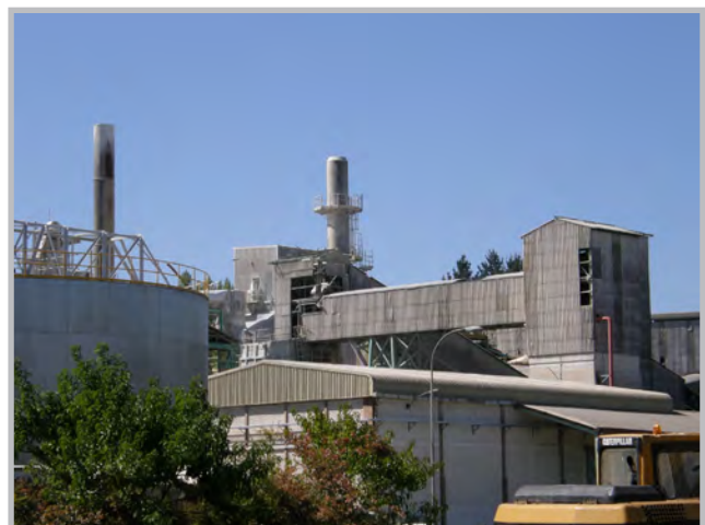
A pulp mill shutdown as a result of the earthquake in Laja, Chile; the plant was awaiting a detailed inspection before resuming operations (Source: RMS)
