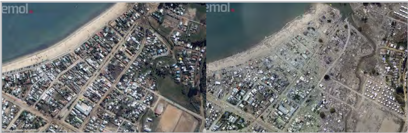
Aerial view of the city of Dichato before the tsunami waves (left) and after the tsunami waves (right), illustrating the complete destruction of buildings in their path (Source: http://www.emol.com/especiales/2010/fotos_AD/terremoto_antesydespues/index.htm )
