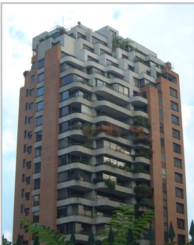
Tall reinforced concrete shear wall building in the comuna of Las Condes in Metropolitan Santiago, Chile, a typical apartment building in region impacted by the 2010 Maule, Chile Earthquake (Source: RMS)
