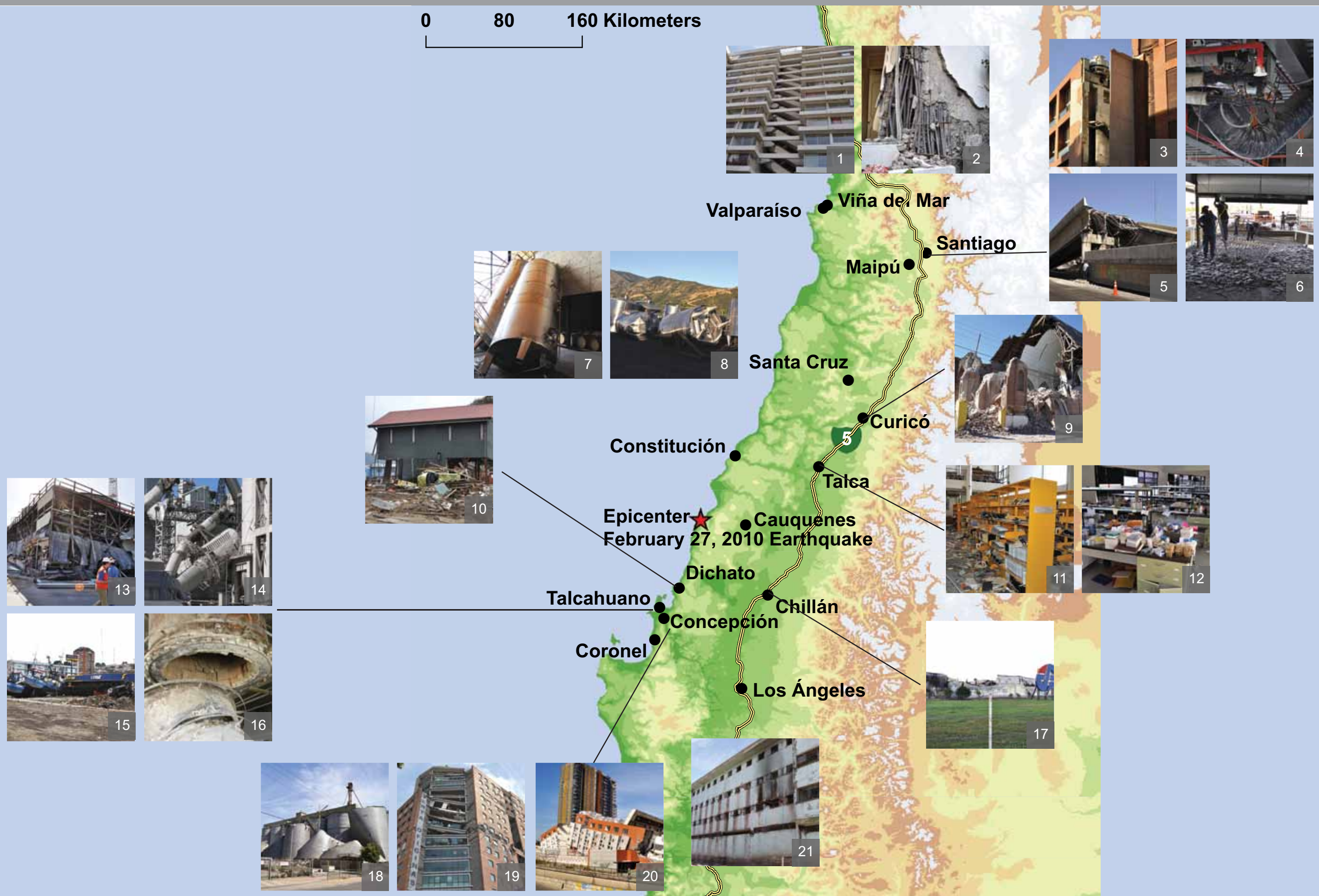
Damage across the impacted region of central Chile, as captured by the RMS reconnaissance teams: (1) the 14-story Edificio Festival in Viña del Mar, built in 1978, suffered severe damage to the stairwells that span two sections of the building; (2) the end of this shear wall in the Edificio Festival ruptured under high compression loads and revealed an abundance of longitudinal reinforcement with little shear reinforcement; (3) buildings in the Huechuraba comuna of Santiago suffered heavy damage as a result of ground motion amplification in the basin; (4) the fire sprinklers at Santiago's International Airport released water over the main terminal; sprinkler systems contributed to contents and business interruption losses throughout the affected area; (5) a series of freeway overpasses in Santiago collapsed due to inadequate connections at the end supports; commuters were forced to use detours through side streets; (6) pedestrian walkways were on the brink of collapse at the main terminal of Santiago's International Airport; (7) the wine in these two storage tanks was salvageable, but nearly a dozen other tanks at this particular winery suffered total losses when they overturned or ruptured; (8) overturned wine tanks are piled along the property line at this vineyard's warehouse in Santa Cruz; inside, stacks of wine cases were filled with broken glass and spilled wine; (9) the entire front section of this landmark cathedral in Curicó collapsed during the earthquake; historic buildings, including many cathedrals, collapsed as a result of their highly vulnerable unreinforced masonry walls; (10) the first floor of this two-story home was entirely swept away and stuffed with debris when tsunami waves crippled the coastal town of Dichato; (11) at the University of Talca, thousands of books in the university library fell off the shelves and were drenched by the fire sprinkler system; (12) the chemistry lab at the University of Talca suffered heavy contents losses as lab equipment and materials fell off shelves and countertops; (13) the cooling towers at a petroleum refinery collapsed during the ground shaking, contributing to business interruption losses; (14) overturned cooling tower at a cement factory in Talcahuano shut down the plant for several weeks; (15) boats were swept down city streets and crashed into commercial buildings as a result of the tsunami waves in Talcahuano; (16) damaged and misaligned equipment at the cement factory in Talcahuano required months for inspections and repairs; (17) a distribution center in Chillán suffered heavy earthquake damage and subsequently lost an entire warehouse to fire following the earthquake; (18) several grain silos ruptured at a facility in Concepción; (19) the O'Higgins Tower in downtown Concepción suffered local, partial collapses in several locations; the building will have to be demolished; (20) the newly-constructed 15-story Alto Rio building completely overturned during the earthquake; (21) severe damage to a confined masonry detention facility in Los Angeles; attempts at escape by the prisoners were thwarted by guards.
