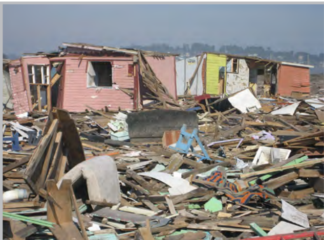
Tsunami damage in Llo-Lleo, Chile, south of San Antonio, following the 2010 Maule, Chile Earthquake (Source: RMS)
