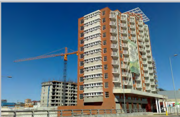
Alto Río building before the 2010 Maule, Chile Earthquake (Source: http://concepcionunderconstruction.blogspot.com/2009/03/edificio-alto-rio-avances-22-2-2009.html )
