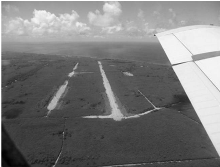
An aerial view of the runway.
