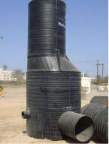
Manhole with mix connections
