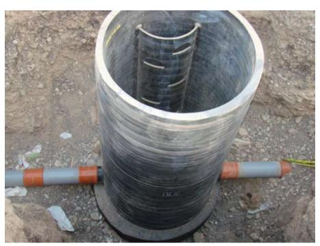
• Manhole with uPVC Pipe Connections
