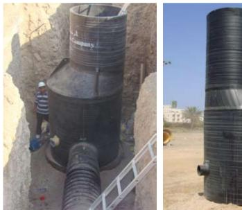
Manhole with Profiled pipes Connections
