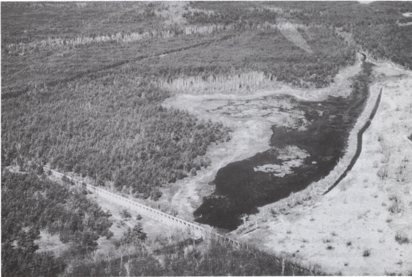
Figure 4. Oblique aerial photograph showing the Million-Dollar Dam and the northwestern flank of Cobblestone Hill (lower right) where it was covered with a concrete veneer to reduce seepage from the former reservoir. The grout-curtain trench can be seen on the right side of the photo.
