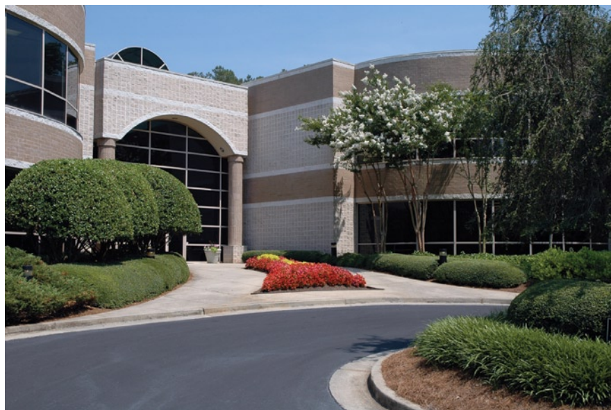
Leica Geosystems' new headquarters building in Atlanta.
