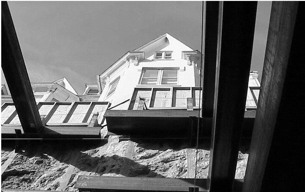
Figure 3. DSM retaining wall supporting adjacent historic structure.
