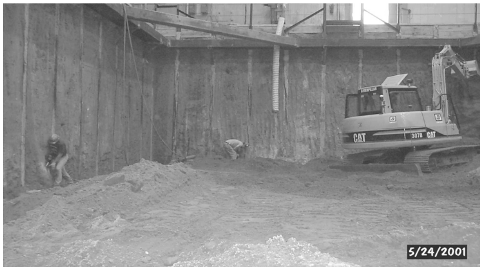
Figure 6. Exposed pit excavation retaining wall/seepage barrier
