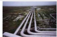
Figure 33: Gas feeder lines at the Yamburg gascondensate field. These pipelines take gas from the wells to the processing plants. Tazovskiy Peninsula, Yamalo-Nenetskiy AO, Russian Federation. Photo taken by Benjamin Seligman, August 1998
