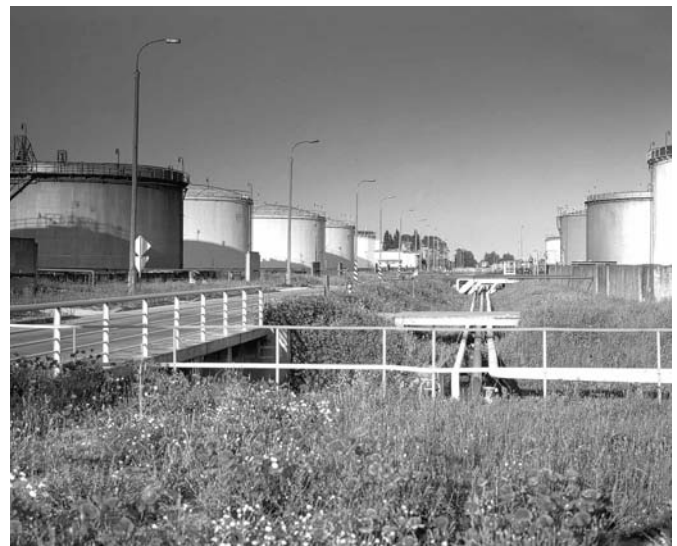
Fig. 23. Typical bulk liquid storage tanks
