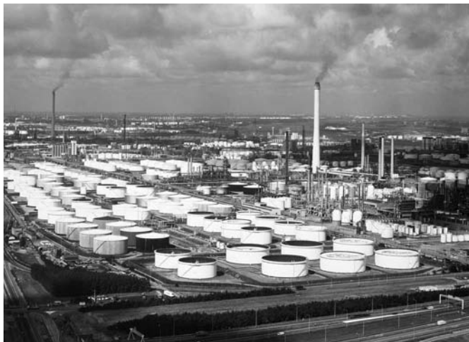
Fig. 1. Refineries make use of bulk storage tanks for which Tank Gauging is essential
