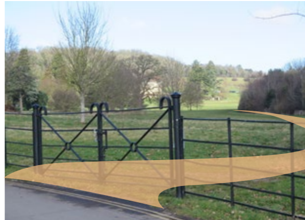
Existing gate off carpark access road. The near gate would be locked open to leave a 1.2m gap
