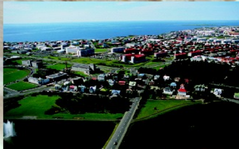
Reykjavik today: "Europe's lung" for its low level of air pollution, now that 99.8% of houses are connected to the geothermal district heating system
