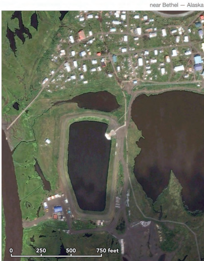
The Kogniginak wastewater lagoon. As in many Y-K Delta villages, separation of sewage from sensitive waterways and wetlands relies on potentially vulnerable earthen structures.
