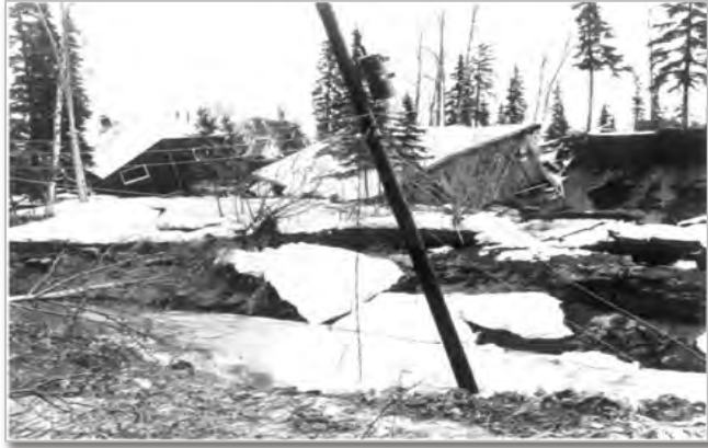
Landslide and slumping effects in the Turnagain Heights area, Anchorage, Alaska, caused by the March 28, 1964, earthquake.
