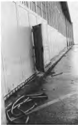
Hangar 1, Buckled Gusset Plate
