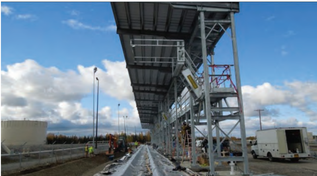
Infrastructure improvements at Eielson AFB include a major rail upgrade to accommodate trains of up to 50 fuel cars delivering one million gallons of fuel per day.
