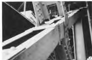
Hangar 1, Buckled Gusset Plate
