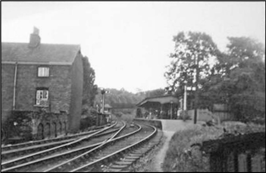
Postcard: the old Stourbridge Town station, since demolished.
