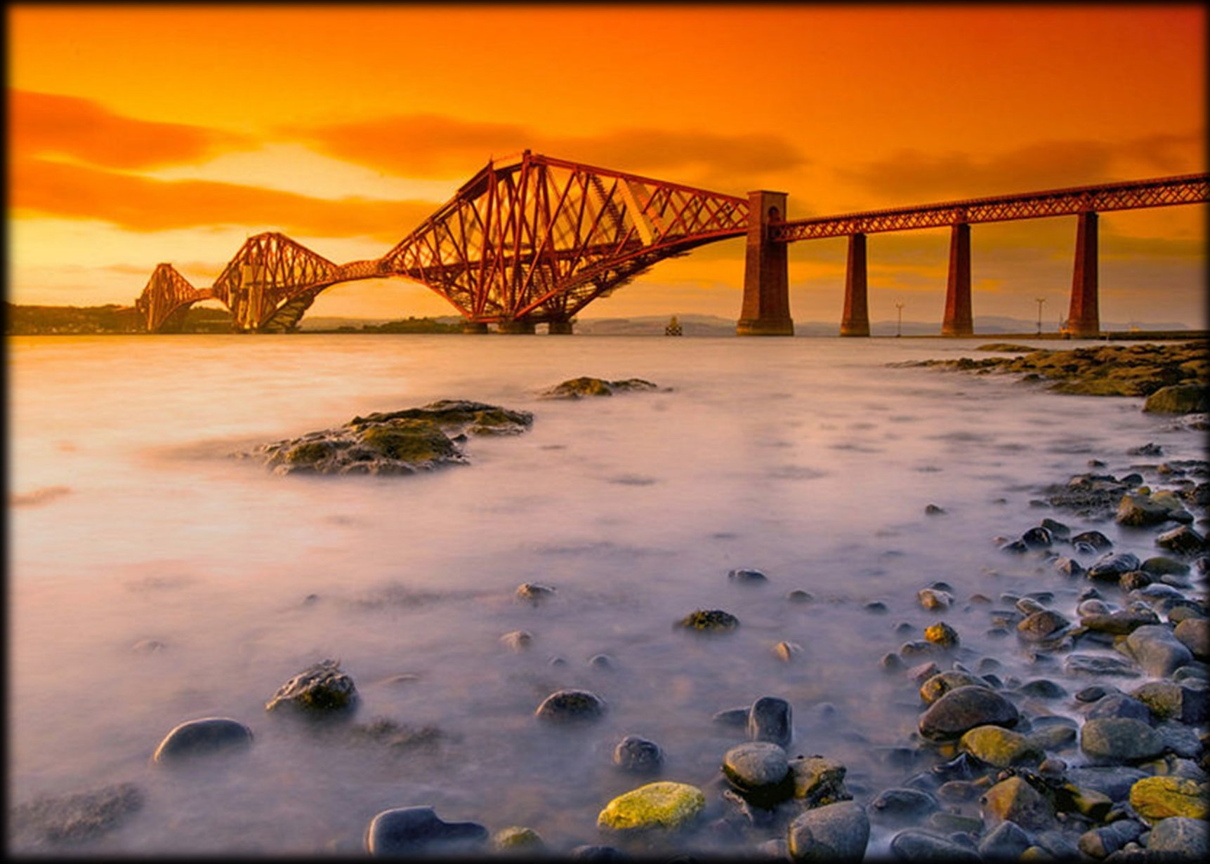
Forth Railway Bridge, Scotland. 1890.
