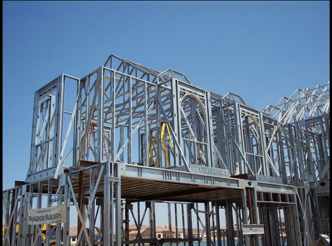
Steel-frame construction.
