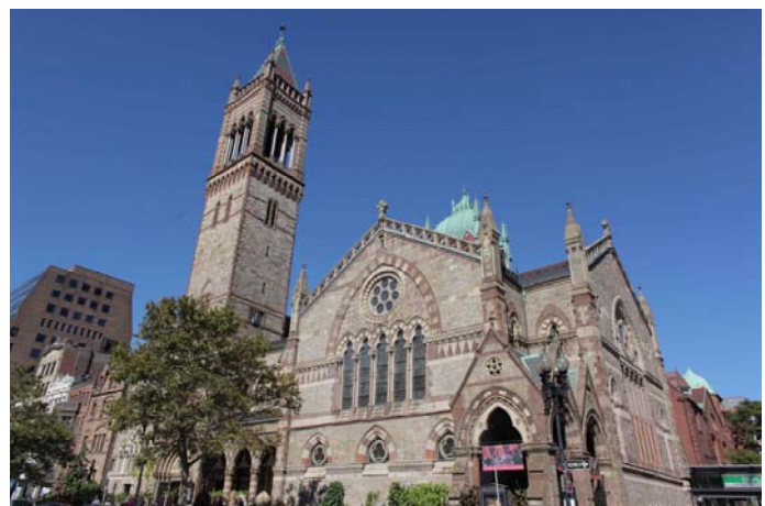
The Old South Church in Boston, Massachusetts Photograph Brian Phillips, Spring 2012
