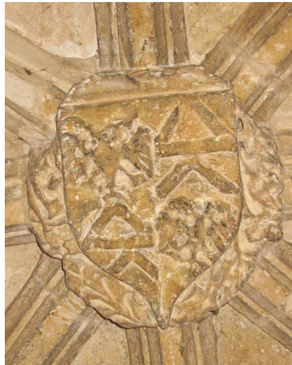
Fig. 12 Arms in the roof of the Porch, St Cyriac's Lacock**
