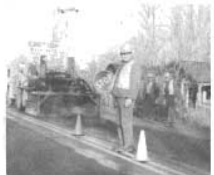
Pavement burning at Fanny Bay on the Island Highway, left to right, W. Lapinski, G. E. Hessel, Burner Foreman, and Harry (Bucket) Waterfield.
