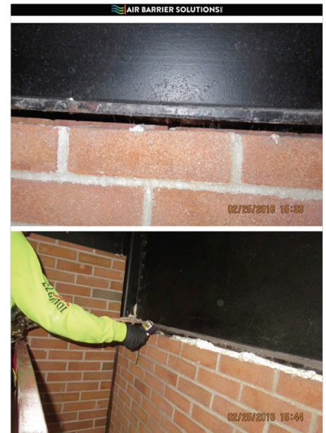
Photo: Air Barrier Solutions
