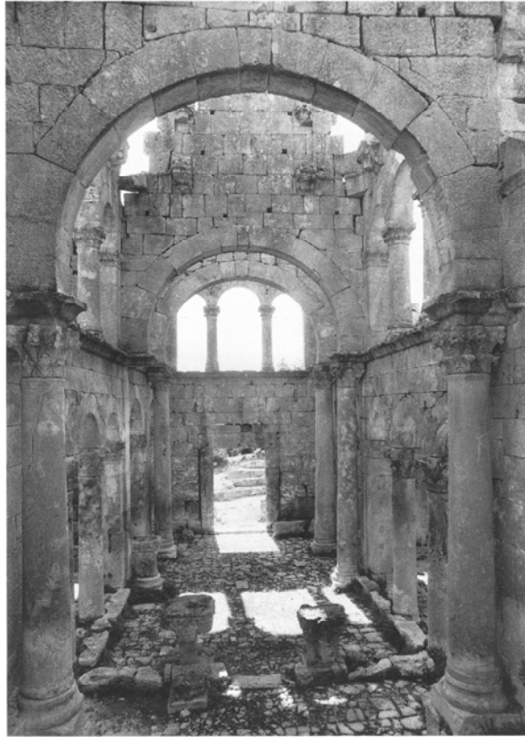
Fig. 12. Transversal arches of the East Church at Alahan Monastir in Cilicia, late 5th century.
