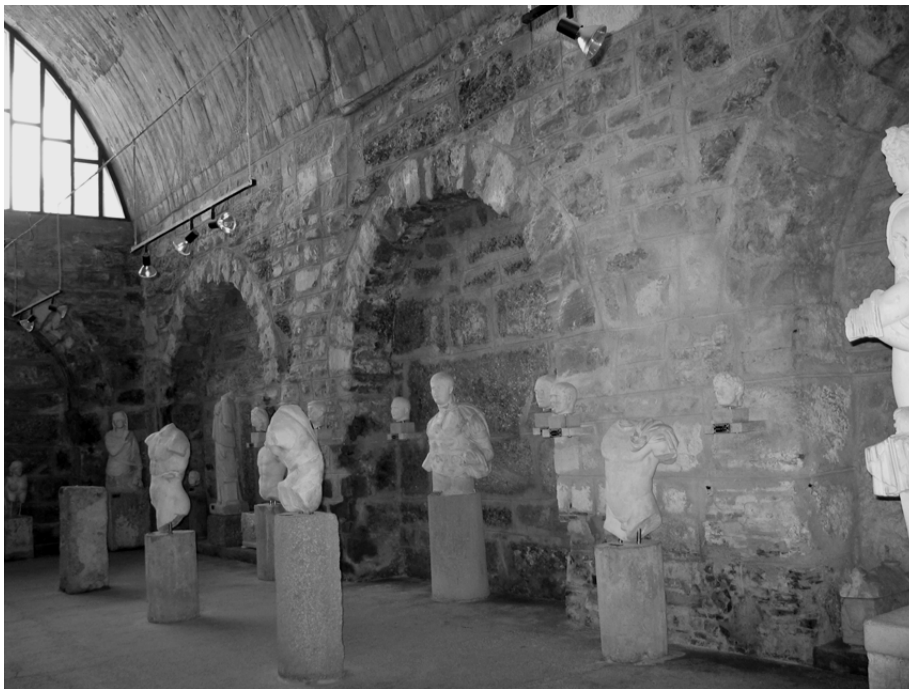
Fig. 11. Blind arcades supported by ashlar pilasters in the Agora Bath at Side in Pamphylia.
