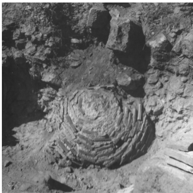
Fig. 13. Byzantine brick cupola found in the Oikoi.
