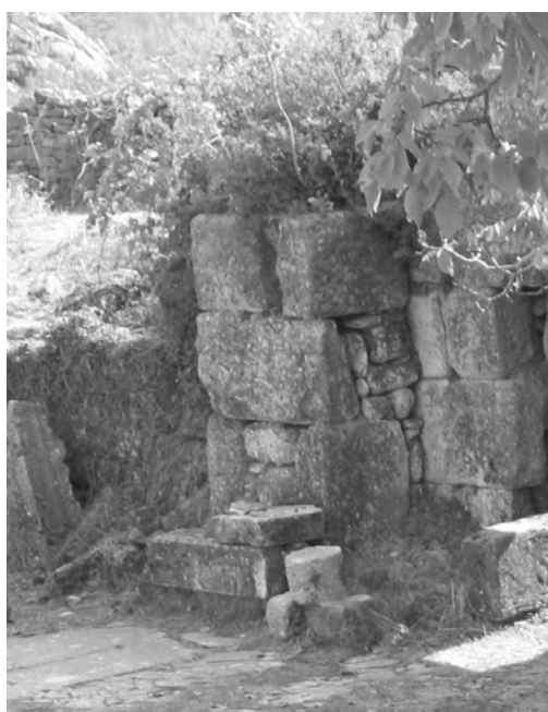
Fig. 7. Pilaster 8 attached to the south wall of Room 4.
