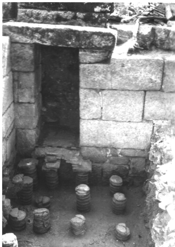
Fig. 10. The hypocaust (Room 9) of the Roman East Bath.
