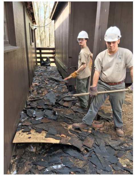
Clearing away old shingles from horse barn renovation
