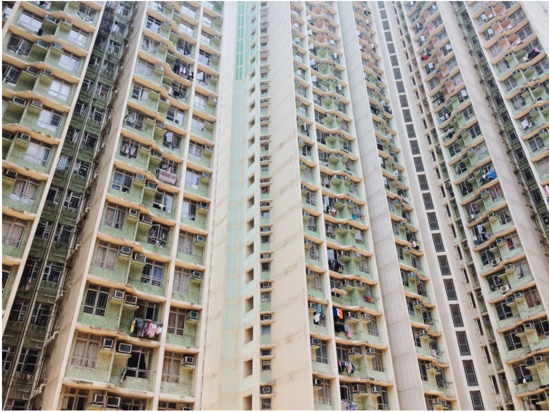
Public Housing flats near Hang Hau Station
