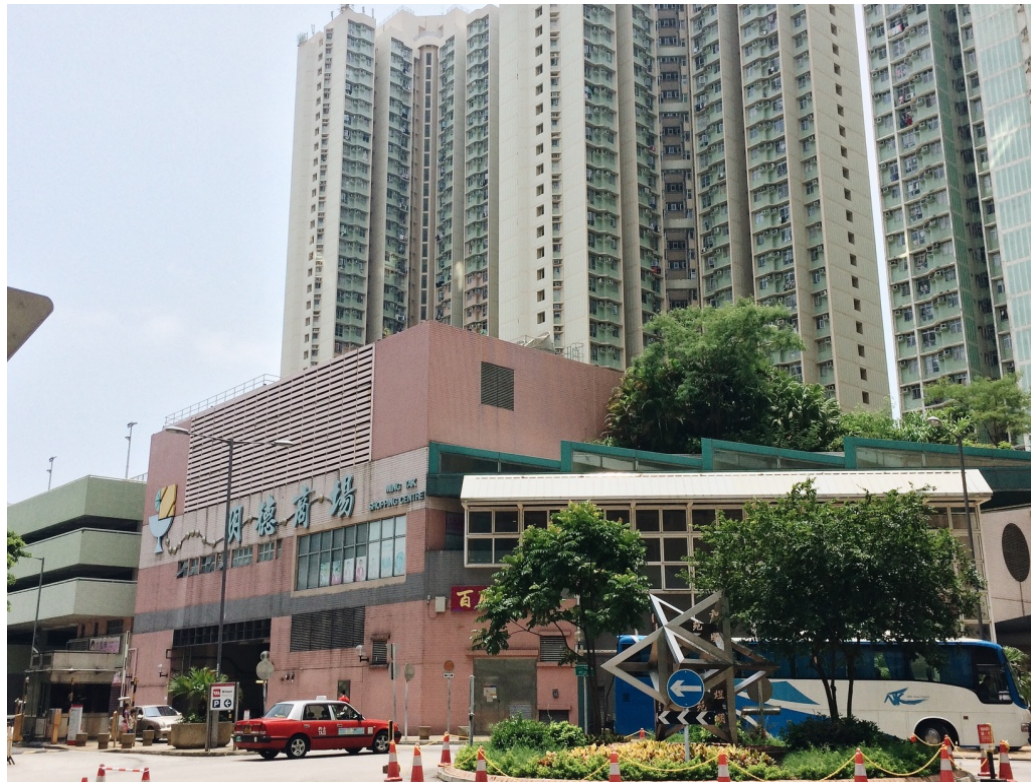
An inoperative supermarket at a public housing estate in Tseung Kwan O
