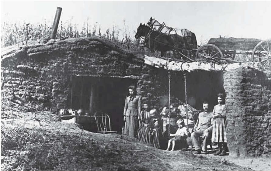
Like these Nebraska homesteaders, many families in the so-called good old days lived in dugouts like this one, made from sod cut from the prairie.
