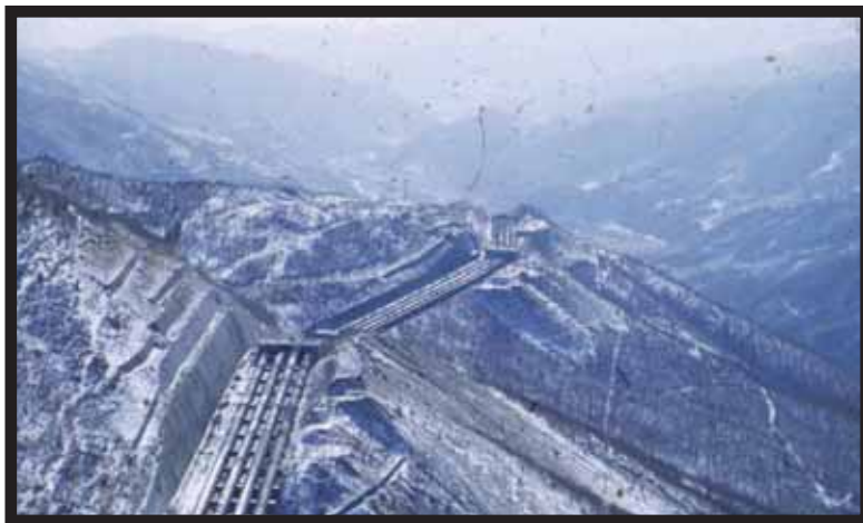
Water pipes carry water from Gatehouse to Power Plant No. 1 far below in the valley at Pojang Station. —Photo by Joseph C. Rodgers
