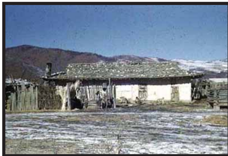
Typical North Korean house at Untaek. Note the stones on the roof to hold down shingles during high wind. Mountains in background were being patrolled by units of the 2/31 Inf., while 3/31 Inf. was further west near the Fusen Reservoir. —Photo by George Rasula
