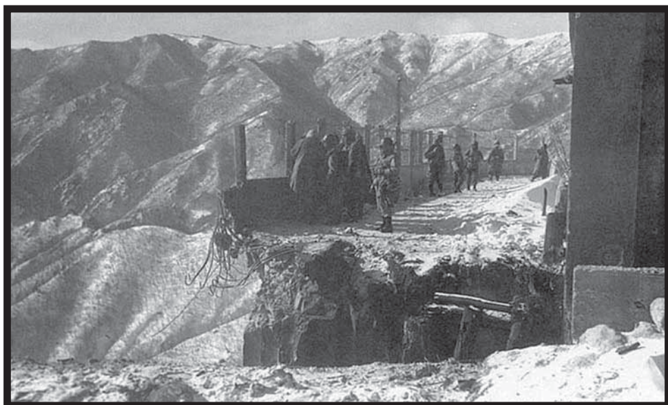
Gateway bridge gap from road level, camera on downhill side. Footpath exists behind building, but no vehicles could use this bridge until repaired by Army and Marine Engineers, spanning gap with sections of a Treadway bridge using equipment of the Army 58th Treadway Bridge Company which was at Koto-ri. —DoD Photo (USMC) A5375
