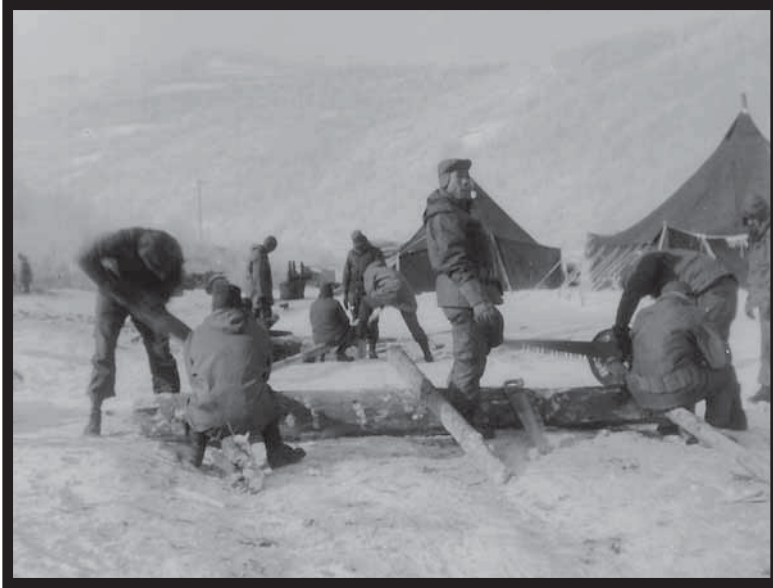
ROK soldiers sawing logs to be used for building weapons positions and bunkers; Koto-ri perimeter. —Courtesy Col. C.W. Guth
