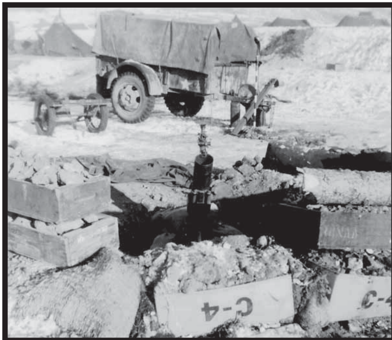
4.2 mortar at Koto-ri. Heavy Mortar Company, 3 Inf. Dug-in emplacement, not too deep as ground was frozen, C-ration boxes full of stones used to build up position. Mortar cart in rear, next to one-ton trailer. Mortar sight on weapon. —Courtesy Col. C.W. Guth
