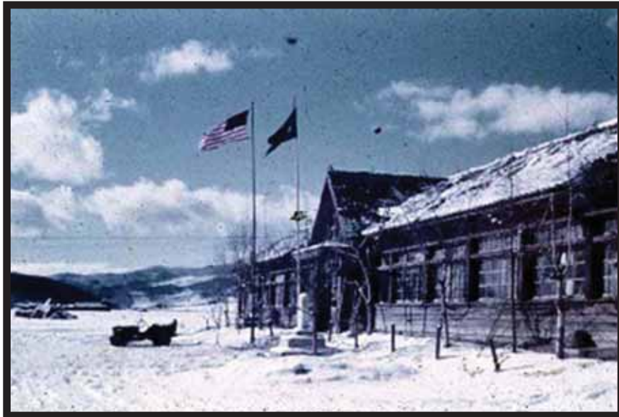
RCT-31 CP in schoolhouse at Untaek, east of the Fusen Reservoir. This is where Dr. Galloway, regimental surgeon, ordered Col. MacLean to bed to get rid of a serious cold saying "Stay in bed or I'll have you evacuated." On 14 November at this location, Chaplain Martin Hoehn's thermometer registered -14 F. Photo by George Rasula
