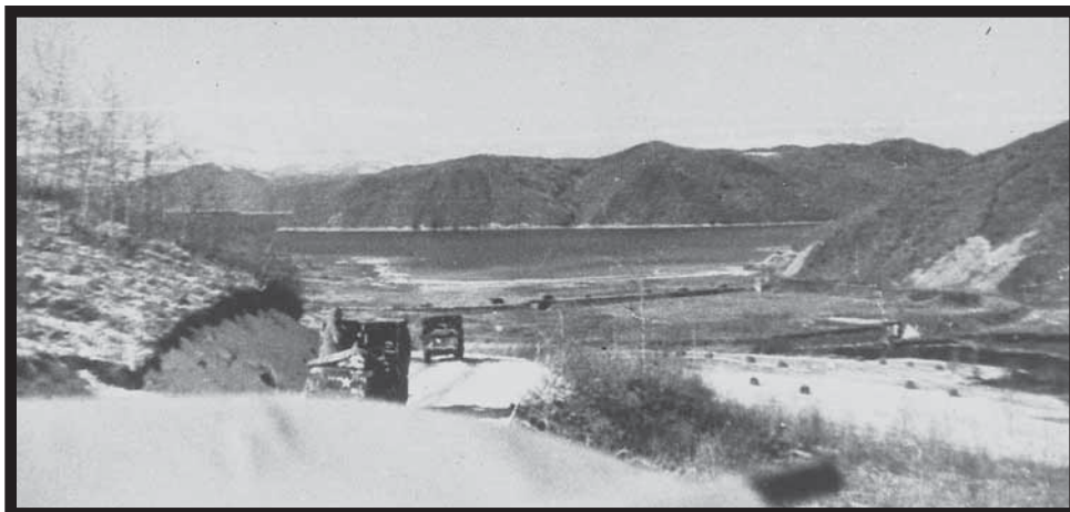
Photo from 5 Marines convoy moving down north side of Hill 1221 on 25 November. Note reservoir in distance is not yet completely frozen. —Source unknown
