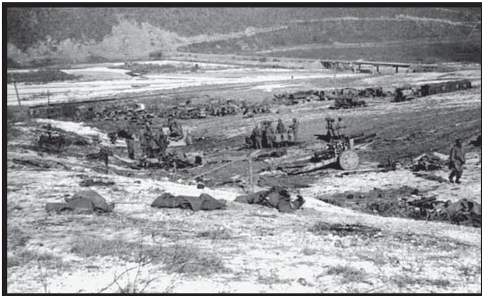
Downhill showing inlet, causeway and bridge. Dead in foreground. Two 105mm. Two clusters of men. Double CP tent at right rear. Many vehicles. [This double CP tent is very near the causeway which was the 3/31 part of the perimeter; tents could be battalion aid station. —Photo by Ivan Long
