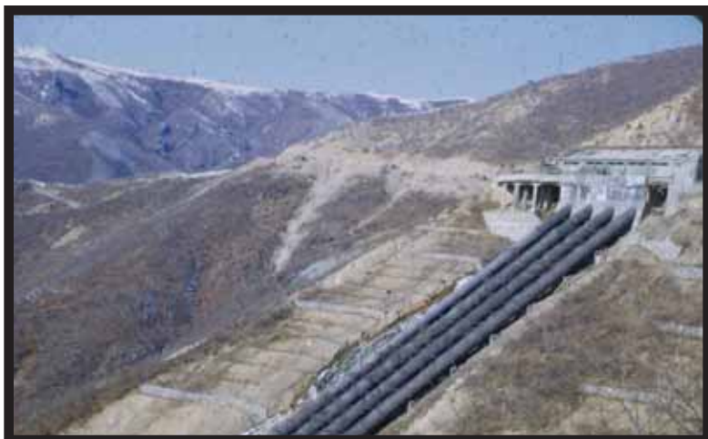
Gatehouse in the Funchilin Pass. Water is controlled from the Changjin Reservoir via a tunnel under the Pass. Normal drainage runs north to the Yalu River. —Photo by Joseph C. Rodgers
