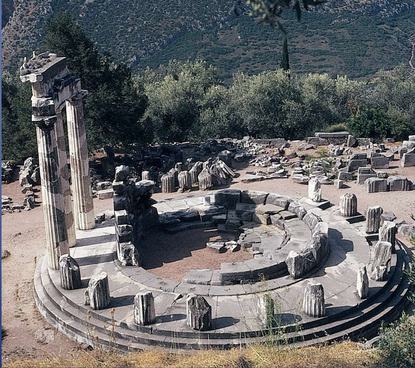
THEODOROS OF PHOKAIA, Tholos, Delphi, Greece, ca. 375 BCE. Outer ring used Doric columns and the inner ring used Corinthian columns.
