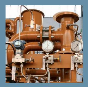
The system supplies oil to machines like compressors, turbines and generators to ensure the proper thermal and physical conditions and cleaning, and providing a stable film of separation between the shaft and the bearing casing under all operating conditions.
