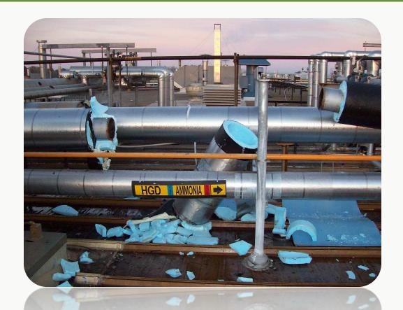
Result of implementing improper sequences of control on a brand new installation along with defective welds and insufficient inspection.
