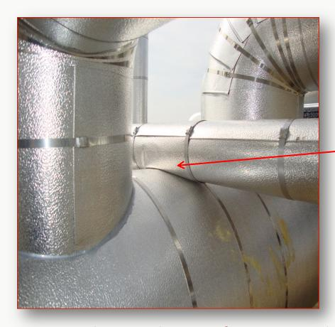
In adequate planning of pipe and insulation routing results in improper installation practices.
